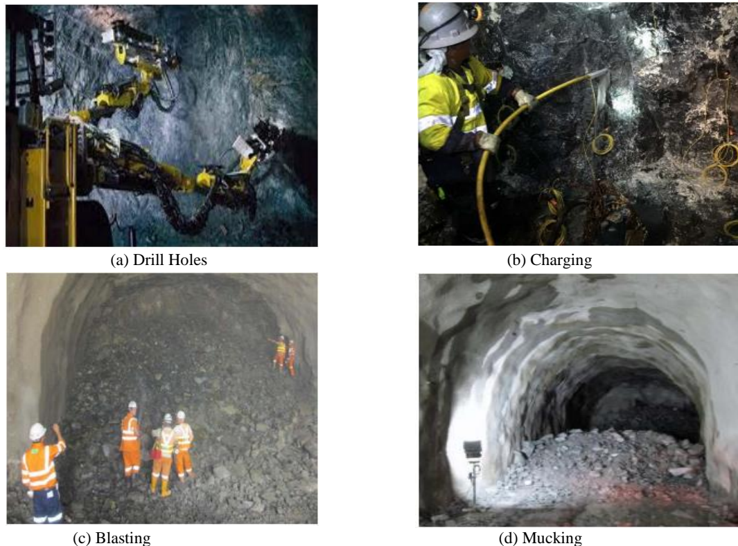
Figure 5: Sequences of NATM [23]. Source: Own elaboration.
